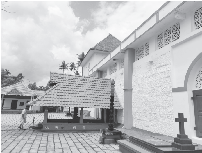
The poomukham at the northern entrance of the church
